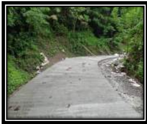
MAT-I (Concreting of 0.211km Access Road with 142 Ln.m Riprap and Grouted Riprap)
